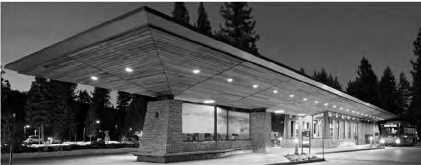
Figure 66 Tahoe City Transit Center [25] (Placer County)
