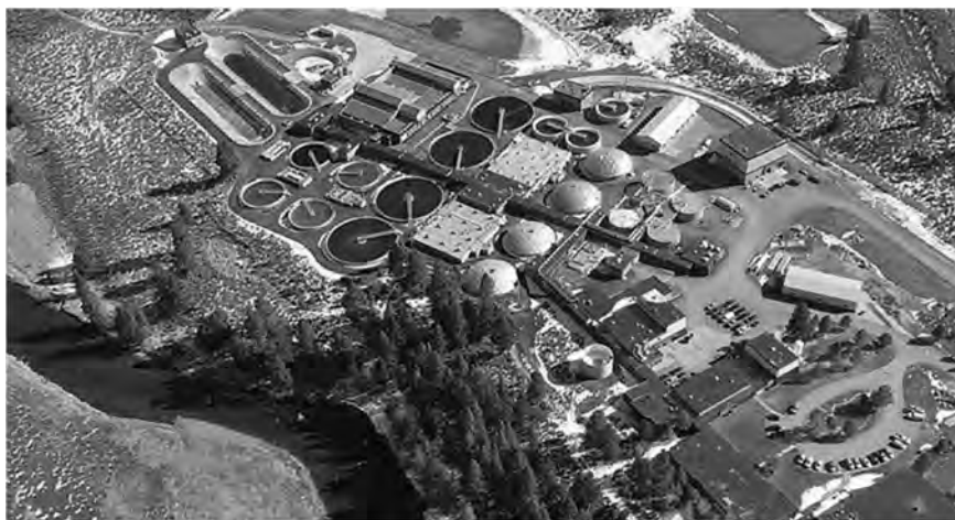
Figure 53 Advanced water reclamation plant constructed by the Tahoe-Truckee Sanitation Agency in 1976-77 for $20 million with the Truckee River shown in the lower-left corner [38]. (TTSA)
