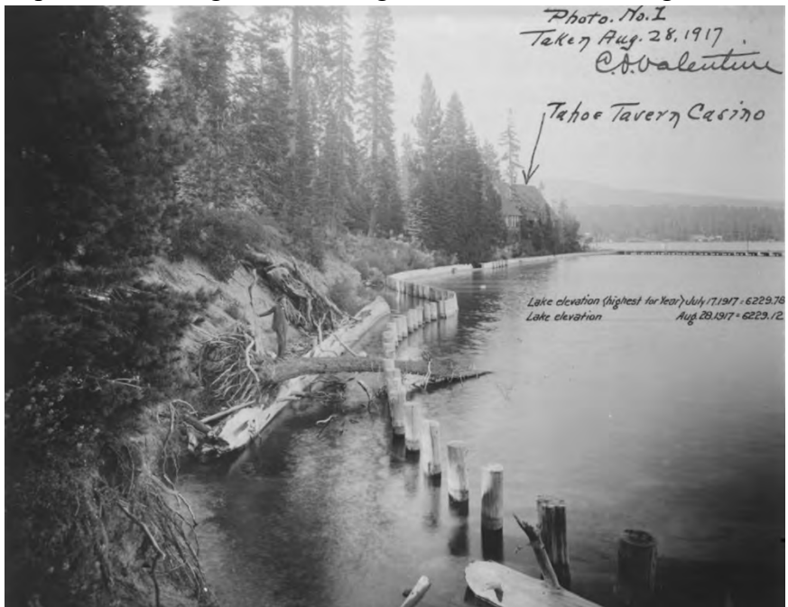
Figure 35 Unnatural shoreline erosion in 1917 near the Tahoe Tavern, Tahoe City [27], caused by the Lake Tahoe Outlet Dam (University of Nevada Special Collections)
